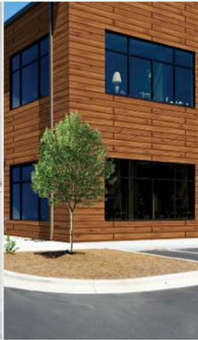
EXTERIOR WALL CLADDING
