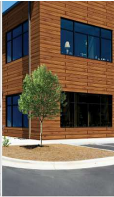
EXTERIOR WALL CLADDING
