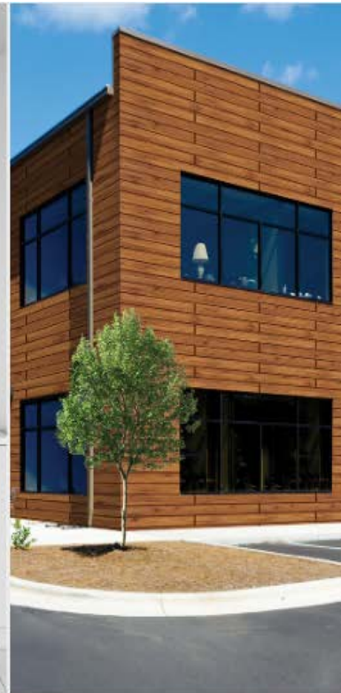
EXTERIOR WALL CLADDING
